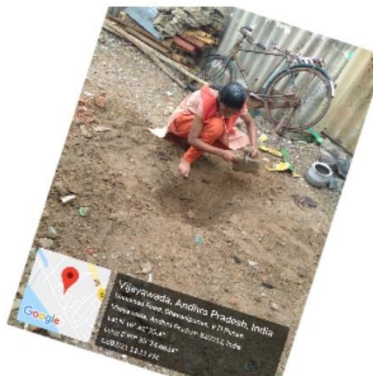
DIGGED PERCOLATION PIT BY BALA KASULU I FMC
